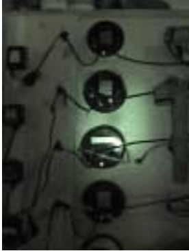
Fig. 4.1 Cox Box in rack
